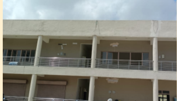
Student Facility Center
